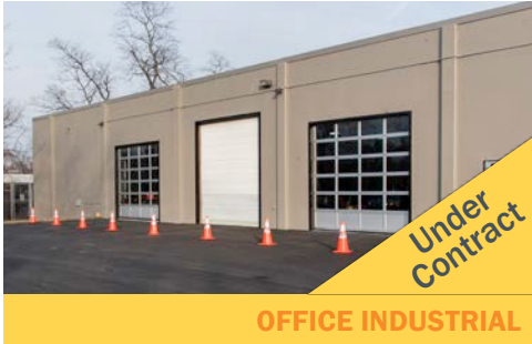
AAA Fleet Facility p. 43
