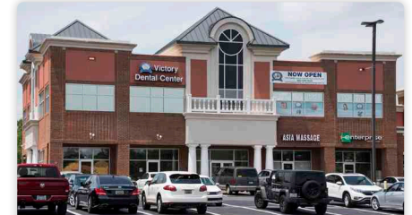
Shoppes at 521 Fort Mill, SC
