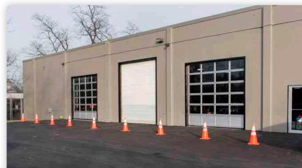
AAA Fleet Facility
