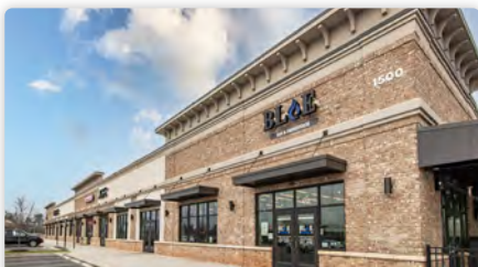
Doby's Bridge Retail
