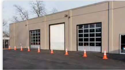
AAA Fleet Facility
