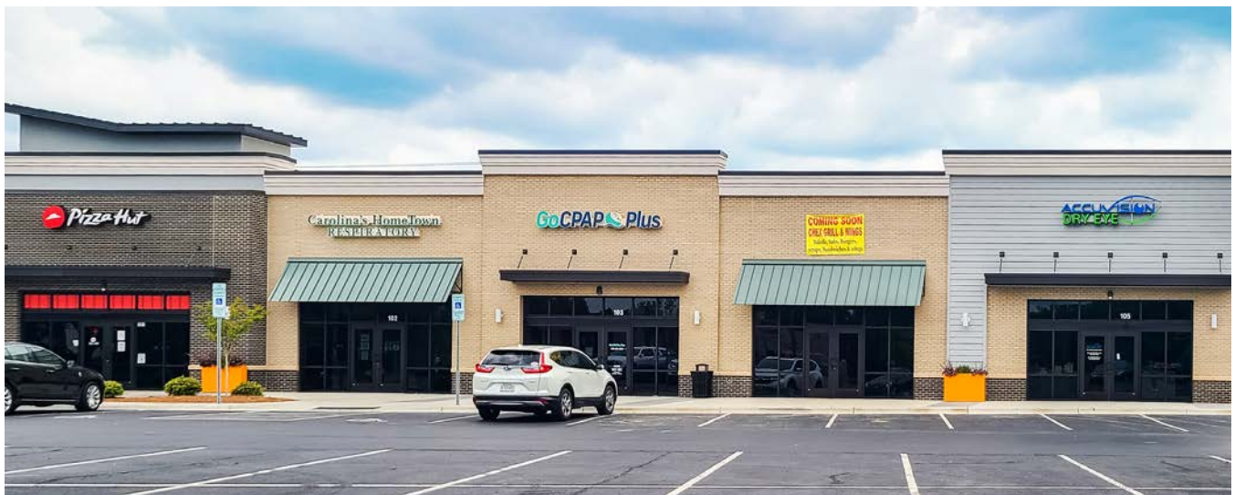
Newly completed outparcel building
