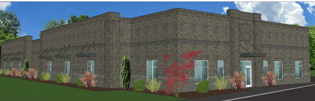
SUITE B ENTRY - BUILDING RIGHT
