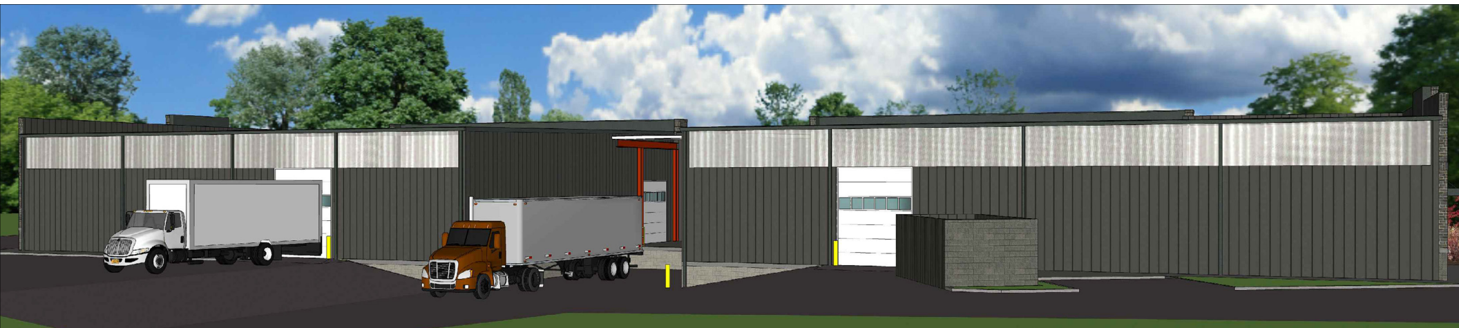
DRIVE-IN & DOCKS - BUILDING REAR
